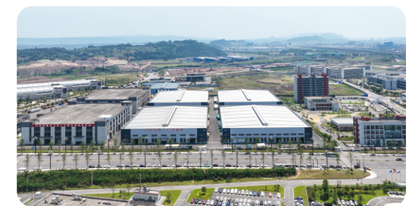
Yibin Industrial Park
